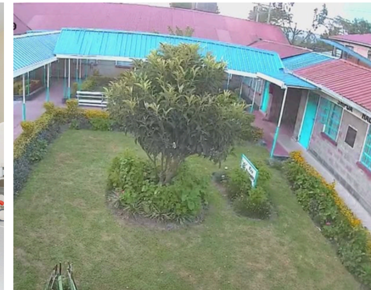
Facility Upgrade at Lanet
