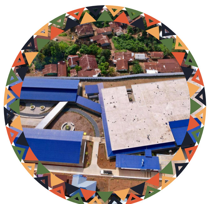
Drone shot of the newly constructed maternal center of excellence in Koidu Town, Kono District. Credit: MoH
