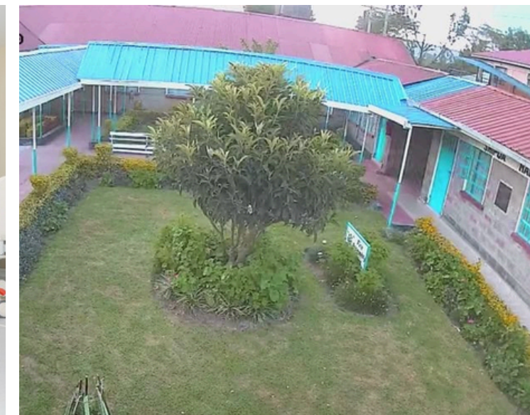
Facility Upgrade at Lanet
