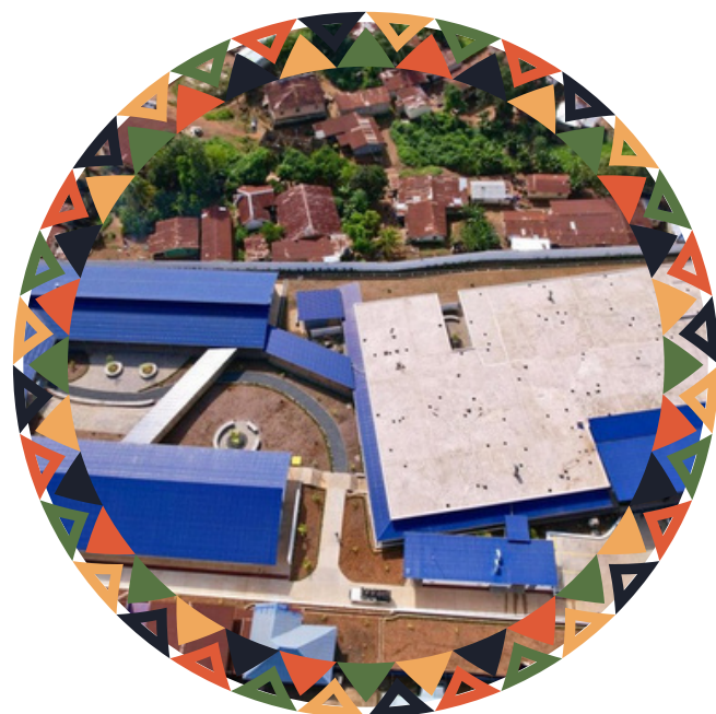
Drone shot of the newly constructed maternal center of excellence in Koidu Town, Kono District. Credit: MoH
